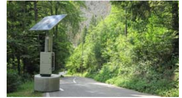
System-Voltage: 230 V AC | Photovoltaics: 390 Wp | Battery: 5 kWh | Inverter: 200 W | Location: Solothurn - Switzerland
