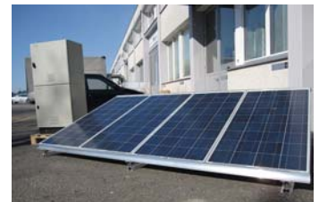
System-Voltage: 230 V AC | Photovoltaics: 540 Wp | Battery: 5 kWh | Inverter: 1600 W | with UPS | Batterie Charger: 0 – 37 A | Location: El Hierro - Spain
